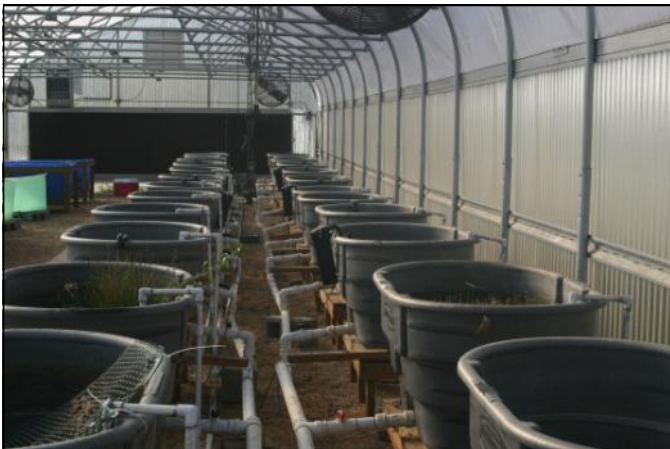
Figure 2. Twenty-four 150-gallon tanks are used for experiments and holding samples of aquatic plants in the aquatic plant greenhouse.
