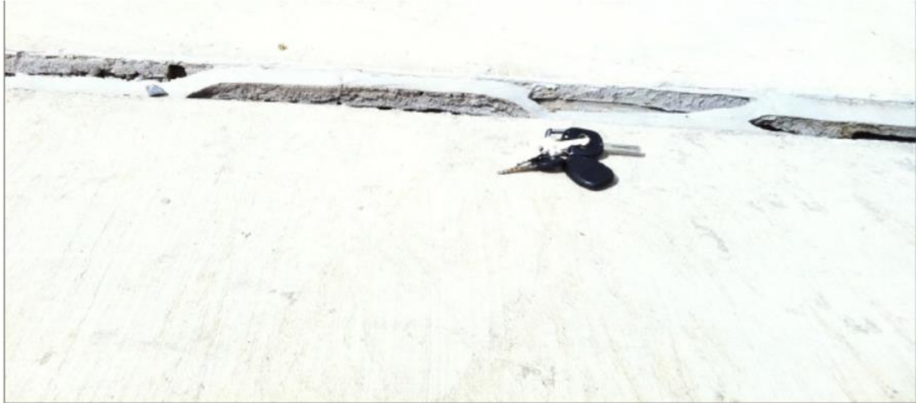
Figure 4. Differential settlement at transition between T-Wall for Lake Borgne Closure (background) and earthen Levee for New Orleans east back segment (foreground) - Taken by R. Gilbert on July 16, 2013.
