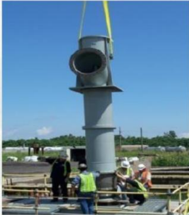
Repair 61 pump stations ($103 Mil)
