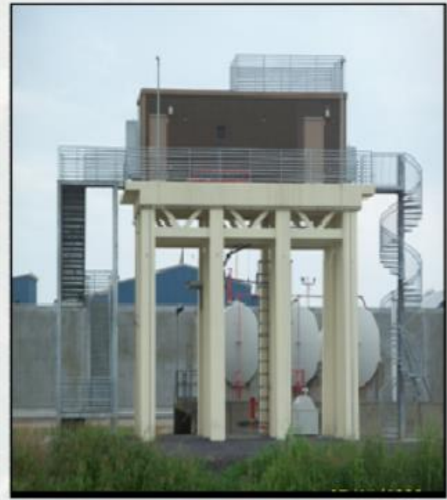
Construct 5 safe houses ($18 Mil)
