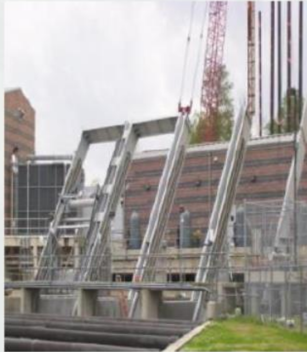
Storm proof 49 pump stations ($322 Mil)
