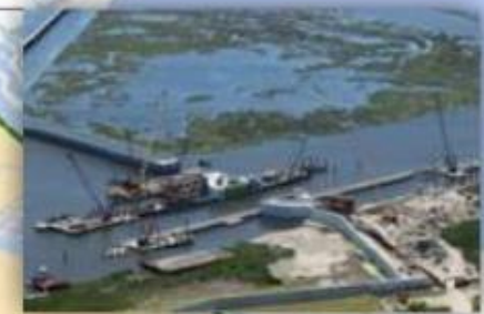
IHNC Surge Barrier
