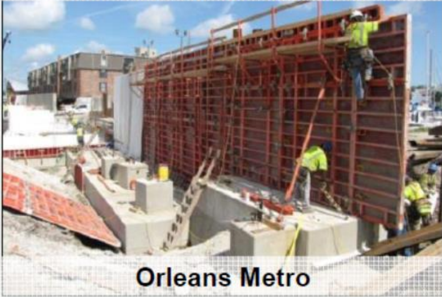
Higher Floodwalls and Levees
