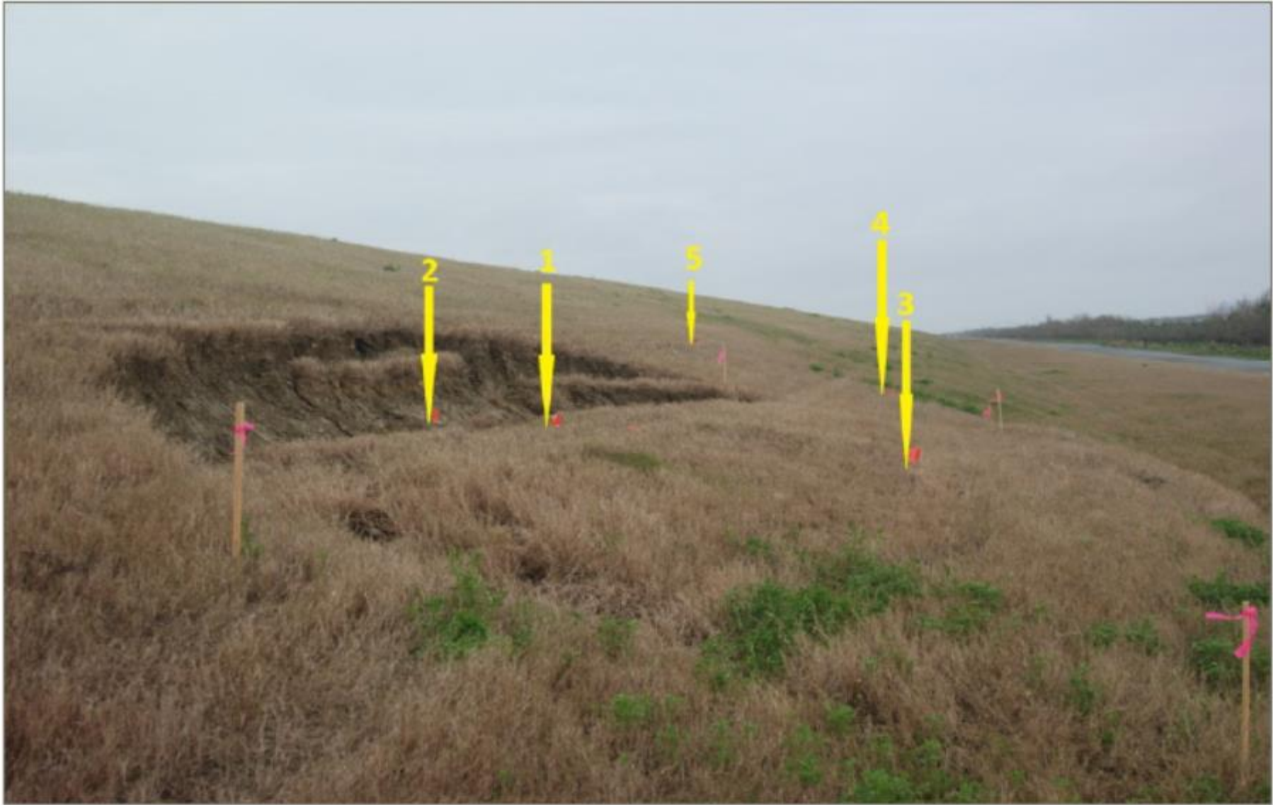
Figure 5. Shallow slope failure near toe of earthen levee for New Orleans east back segment. Numbered arrows indicate sampling locations for a previous study. (Provided by R. Brouillette, CPRA).
