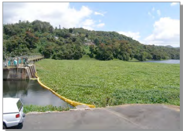
Photo 4 – Water hyacinth clogging a hydroelectric dam on Lake Carraizo, San Jaun, Puerto Rico. Photo by Victor Gonzalez.
